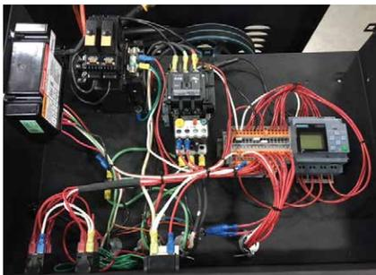
**PROGRAMMABLE SMART CONTROL** now standard for all VNG machines allows auto start/stop and time delay shutdown features without changing any hardware. It also provides complete control of the equipment run time.
